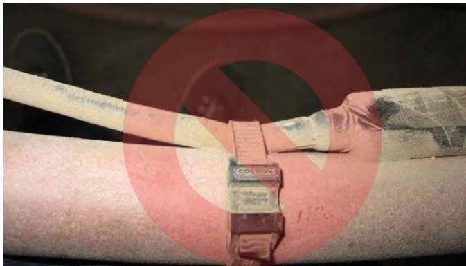
Figure 3. Do not use Zip-Ties Directly on Cables
